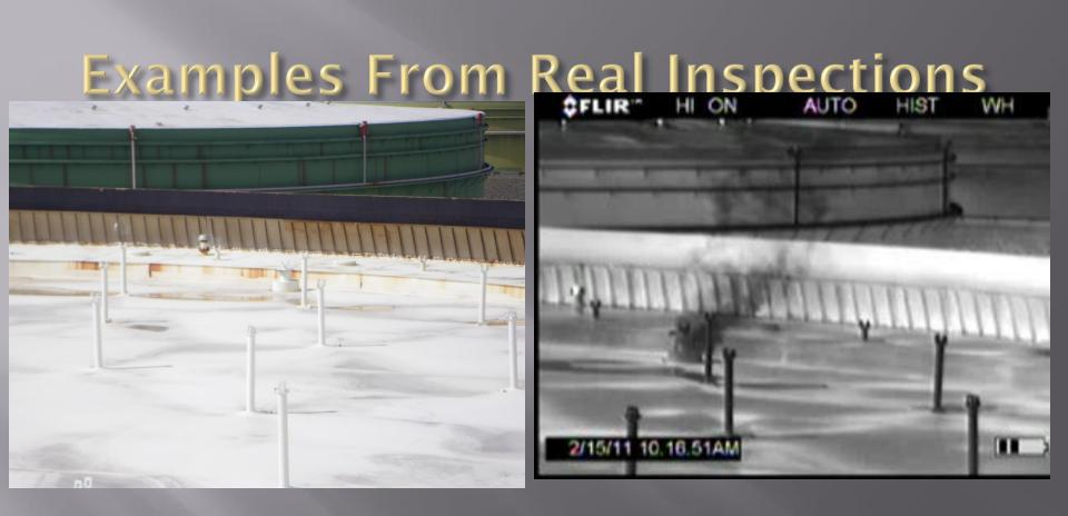
Storage vessel bleeder vents must be closed at all times unless the tank roof is being landed or floated off the leg supports
