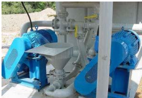
Hopper to Mix Mud
