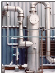
Venturi Scrubbers are used to remove very fine dust, mist and can also remove gases.
