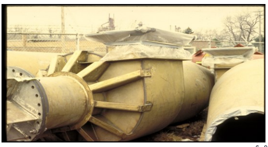
Cyclones Staged for Installation in a Fluid Catalytic Cracker (FCC) Regenerator
