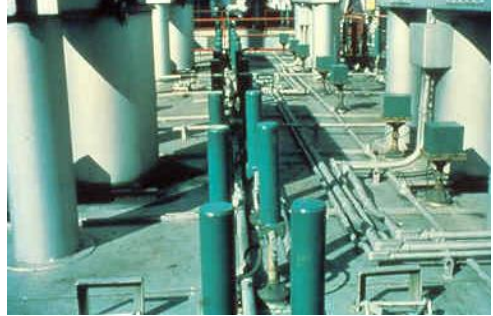
A current pulse raises the steel plunger inside the MIGI rapper then, by the effect of gravity, the plunger drops back and strikes a rod which is connect to many plates inside the ESP.
