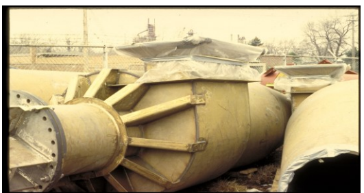
Cyclones Staged for Installation in a Fluid Catalytic Cracker (FCC) Regenerator
