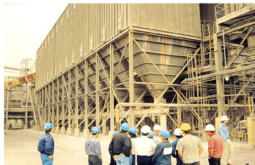
16-compartment baghouse used at tail end of Portland Cement processing plant.
