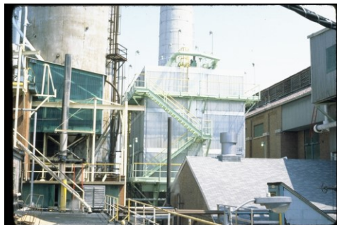
Reverse Air Baghouse Controlling an Industrial Coal-Fired Boiler
