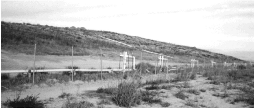
Figure 3-5. Abandoned Horizontal Barrier Trench System.
