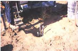
Installation of a Three Tier Probe
