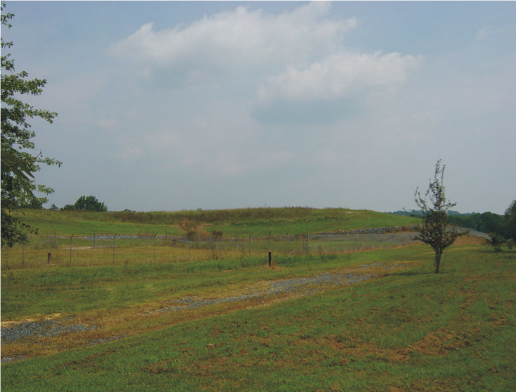
View of the Bush Valley Landfill
