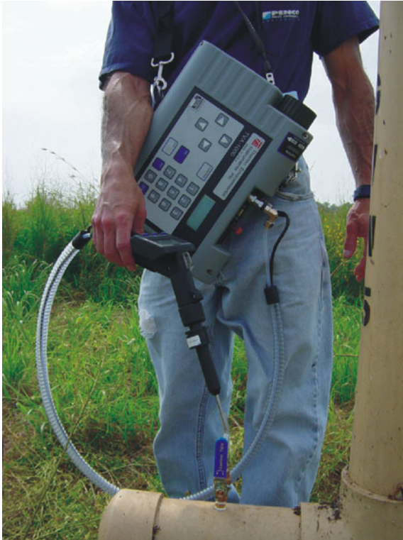
Landfill Gas Screening at a Passive Vent
